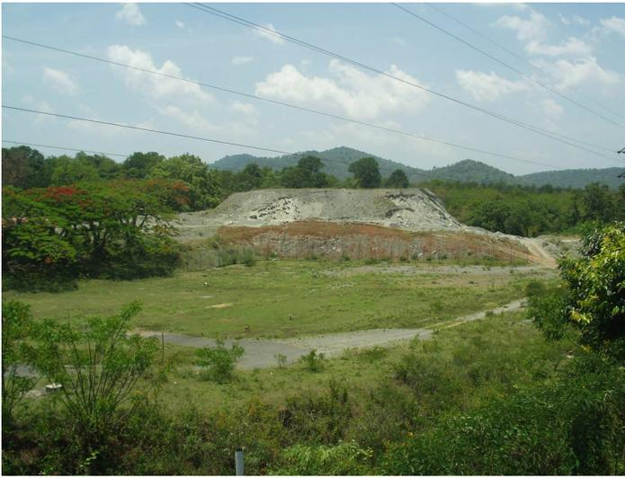
The construction phase requires the removal of the rock excavated from the tunnel and laboratory. The recommended plan is to store the muck (mainly granite) in the existing dumping yard created for the power project which is located near the portal. Hence truck movement is restricted to a small region within the TNEB-owned land.
