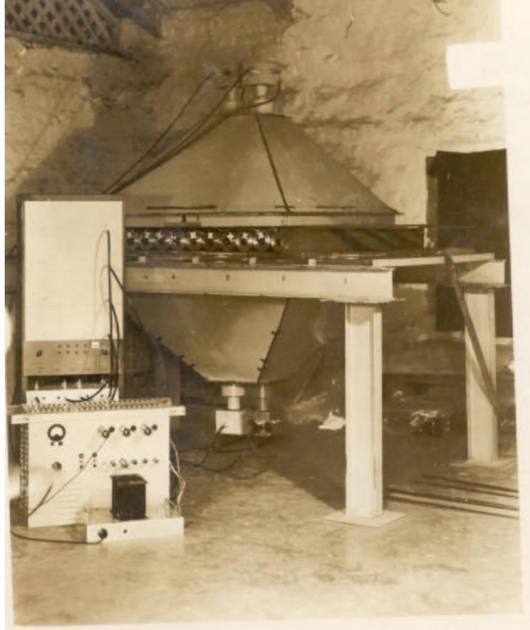
Fig. 1 The scintillator-lead-GM counter telescope used at great depths in KGF mines. A coincidence of pulses from PMTs viewing the two scintillators and the sandwiched GM counter array provided the signal with negligible background.
