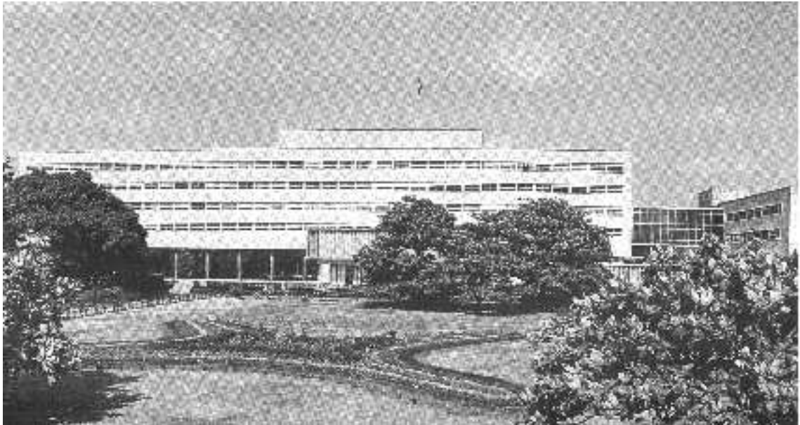
Figure 3.1: View of the Tata Institute of Fundamental Research, Bombay.
